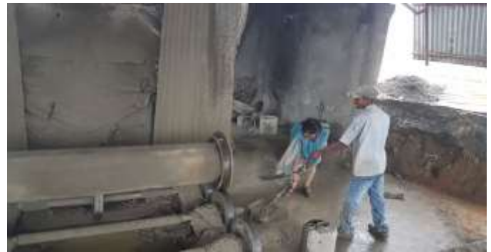
Figure-1 Casting of pipe
