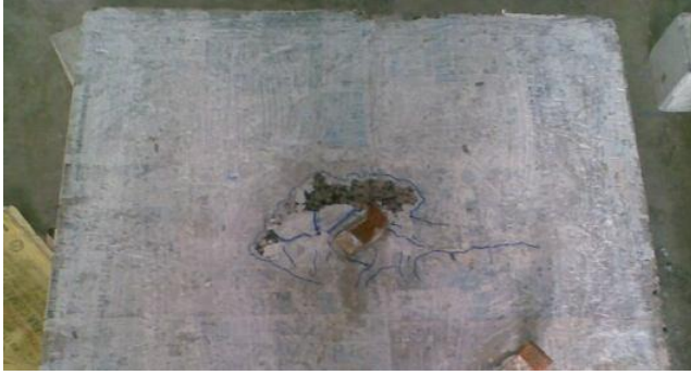
Fig.2 : Fiber reinforced geo-polymer concrete slab
