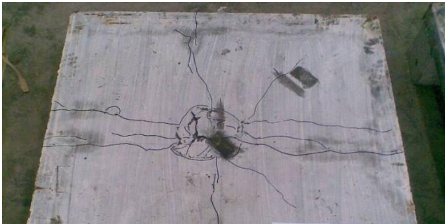
Fig.3 : Fiber reinforced ordinary Portland cement concrete slab
